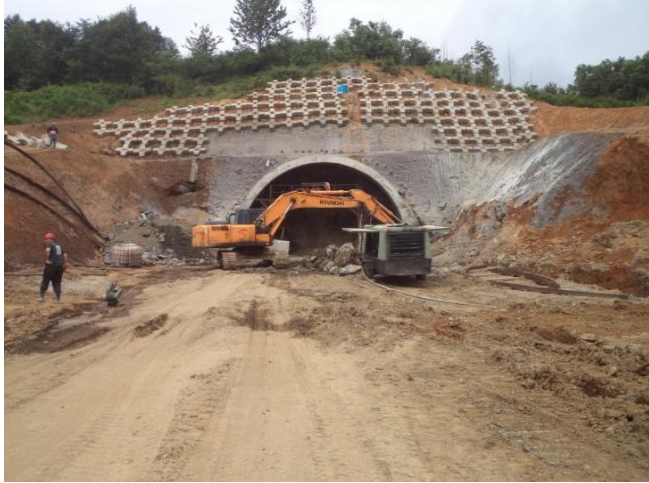
Photo 13: Monitoring of Tunnel Construction works
