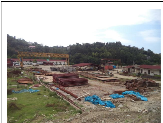
Photo 8: Scrap material scattered at the campsite
