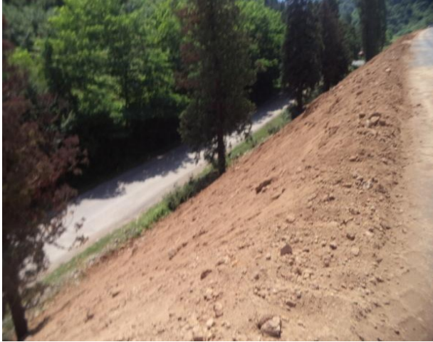
Photo 11: Slopes to be covered with top soil
