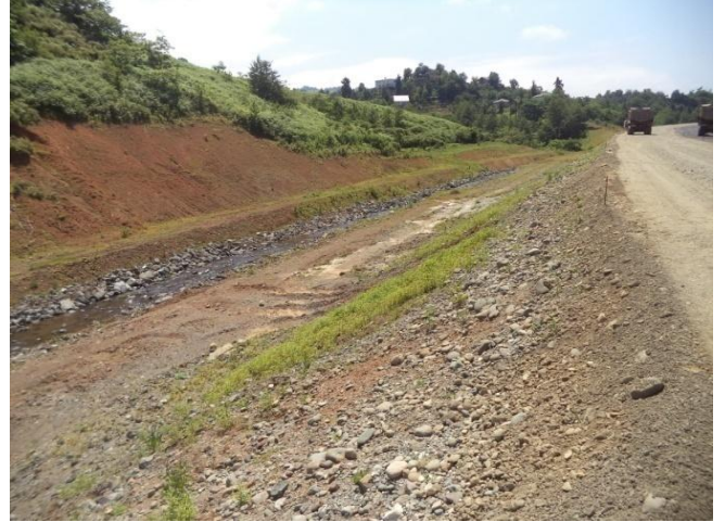
Photo 12: Slopes to be covered with top soil
