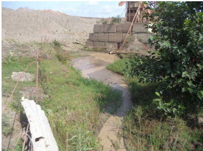
Photo 6: Basin of crushing plant full of silt
