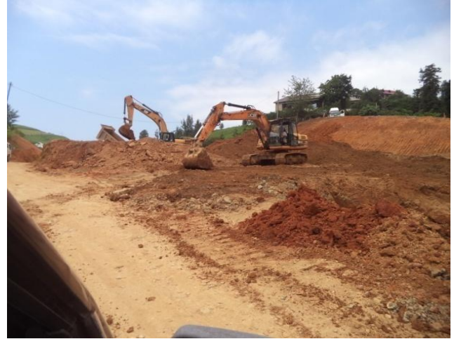
Photo 14: Monitoring of slope cut and earthworks
